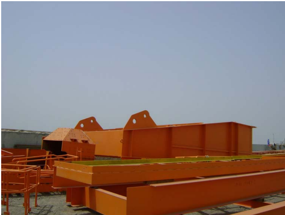
Fig. 6: Stacker cum Reclaimer-1 Materials stocked near its foundation (BC-03)
