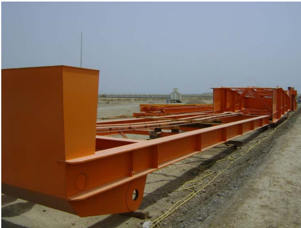
Fig. 8: Stacker cum Reclaimer-1 Materials stocked near its foundation (BC-03)
