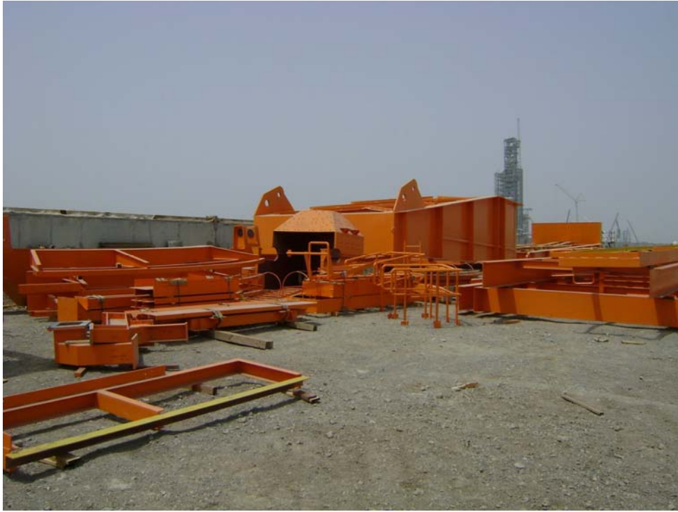
Fig. 5: Stacker cum Reclaimer-1 Materials stocked near its foundation (BC-03)
