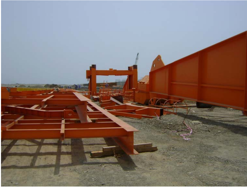
Fig. 7: Stacker cum Reclaimer-1 Materials stocked near its foundation (BC-03)
