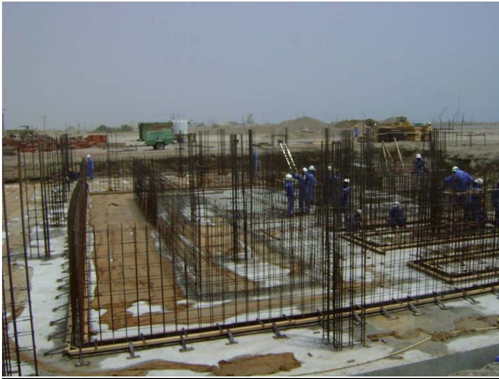
Fig. 17: MHSS-1, Trench work in progress
