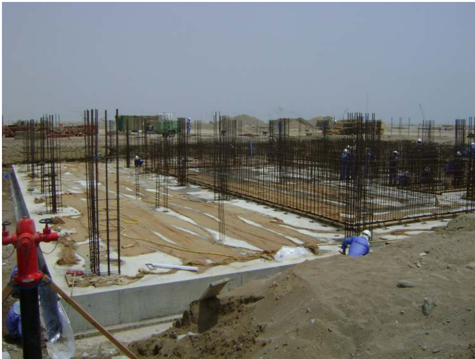
Fig. 16: MHSS-1 (Material Handling Sub Station-1) RCC Completed
