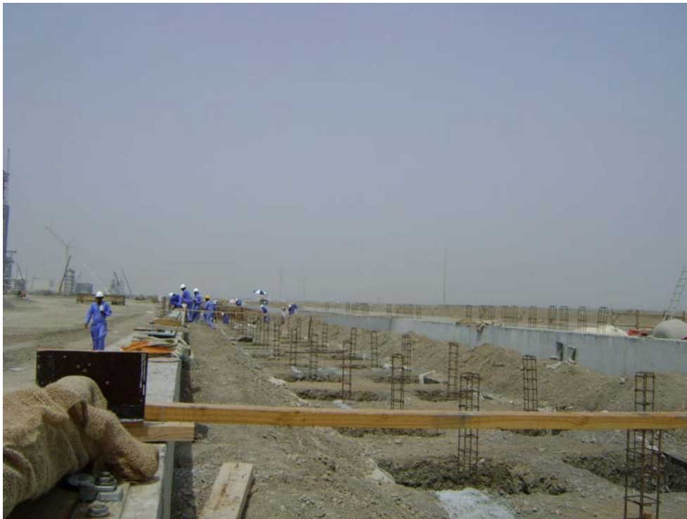
Fig. 10: W.I.P. on remaining Pedestal of Conveyor no. BC-03
