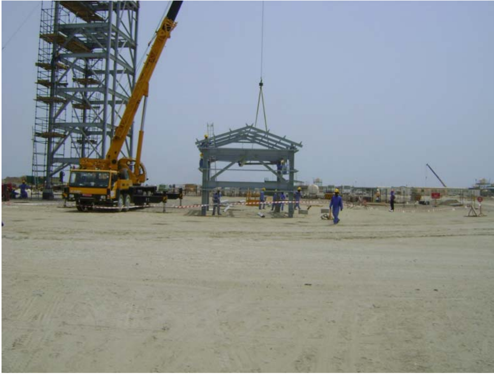
Fig. 13: Canopy of TT-04 (Assembled at ground & ready to commission)
