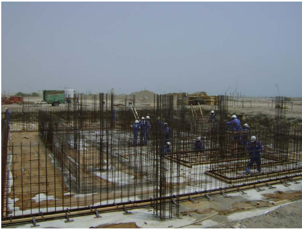
Fig. 18: MHSS-1, Trench for Cables on fast track
