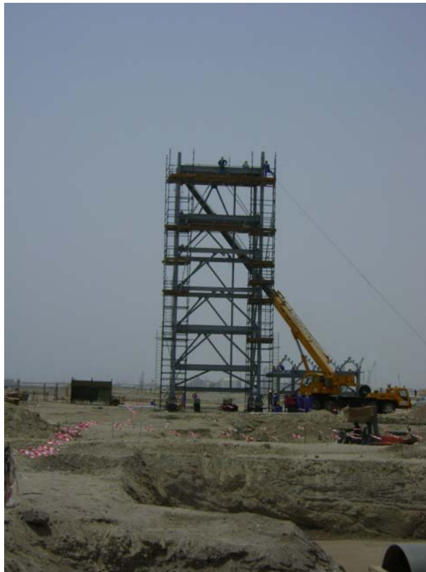
Fig. 12: Transfer Tower, TT-04
